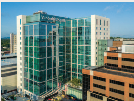
The 495,000-square-foot Jim Ayers Tower on 21st Avenue is the largest facility expansion to date. The tower began welcoming patients in October 2025.
