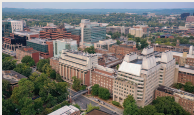
The Vanderbilt Health Main Campus in Nashville has seen extensive growth, including the Jim Ayers Tower and a four-story expansion at Monroe Carell Jr. Children's Hospital at Vanderbilt.
